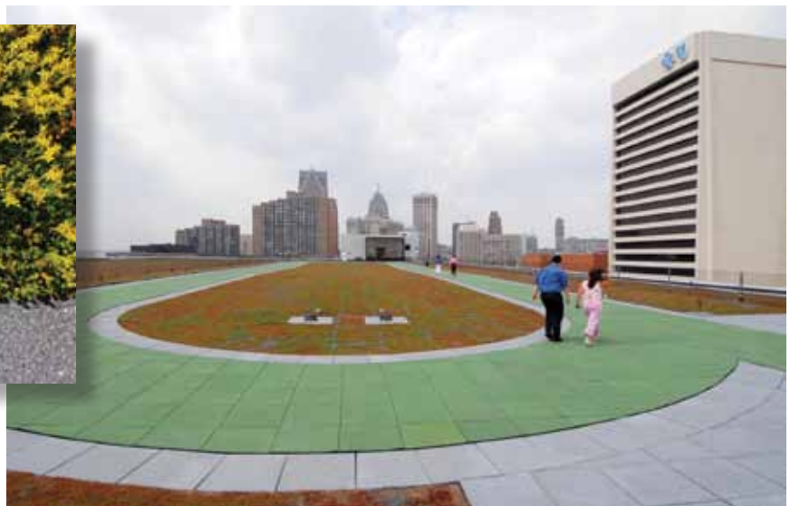
The BCBSM parking structure features eight varieties of low-growing sedum in 2 to 3 inches of growing medium over drainage layers. The saturated weight of the system is approximately 15 psf.
