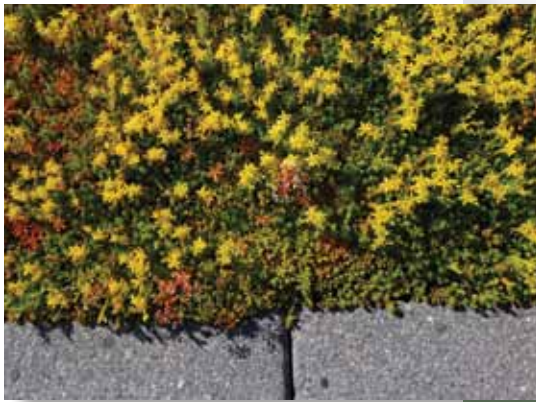
The BCBSM parking structure features eight varieties of low-growing sedum in 2 to 3 inches of growing medium over drainage layers. The saturated weight of the system is approximately 15 psf.
